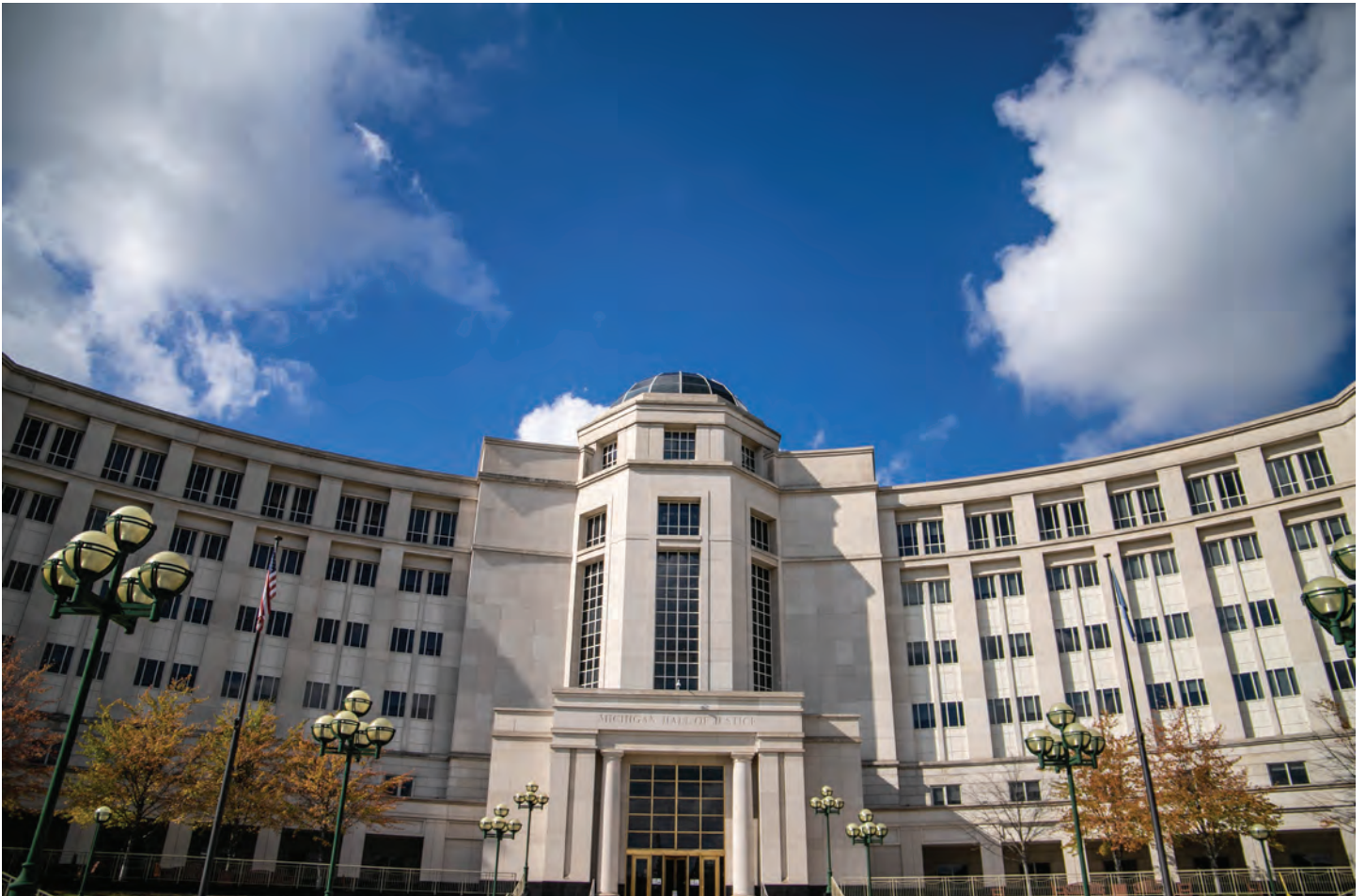
Exterior of Michigan's Hall of Justice. Photo by Sarah Lawrence Brown | State Bar of Michigan.
